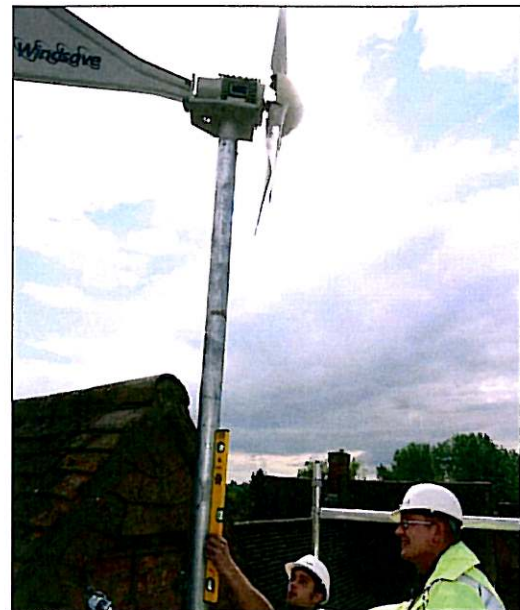
Installation of new wind turbine
