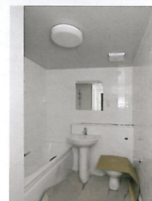
: Pods are positioned against the party walls, rather than being part of the construction, to ensure acoustic targets are met.
